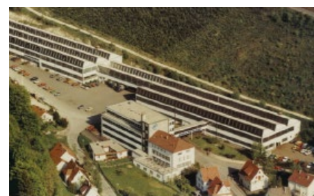
Production building Albstadt
